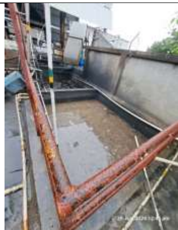
MEE/MVRE Concentrate collection tanks
