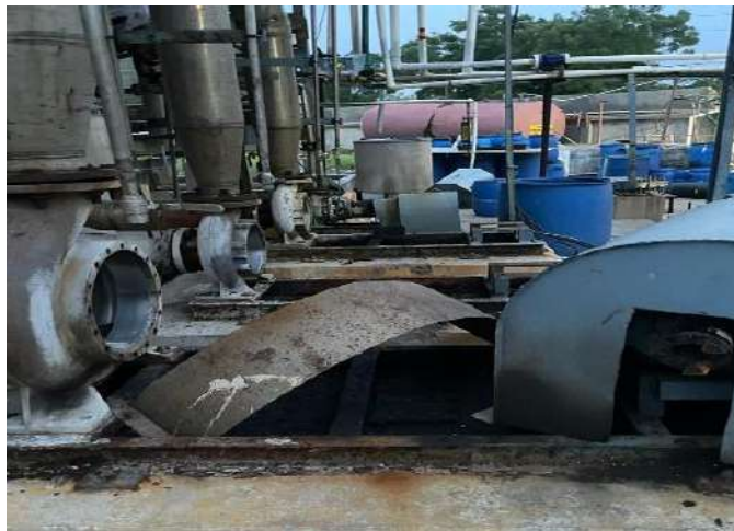
Removal pumps from MEE
