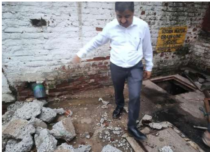
Opening of HDPE pipe from chamber near storm water drain
