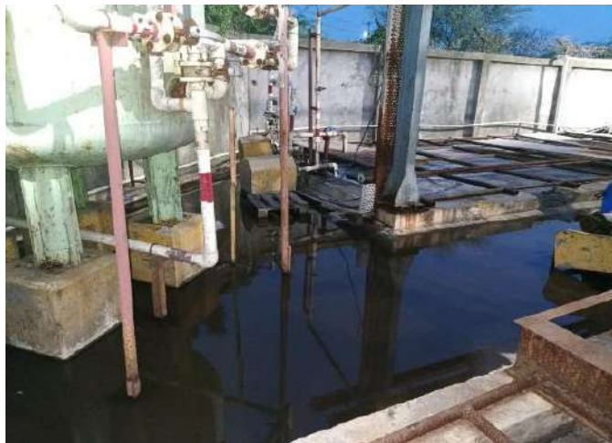
Accumulation of contaminated alkaline water within premises.
