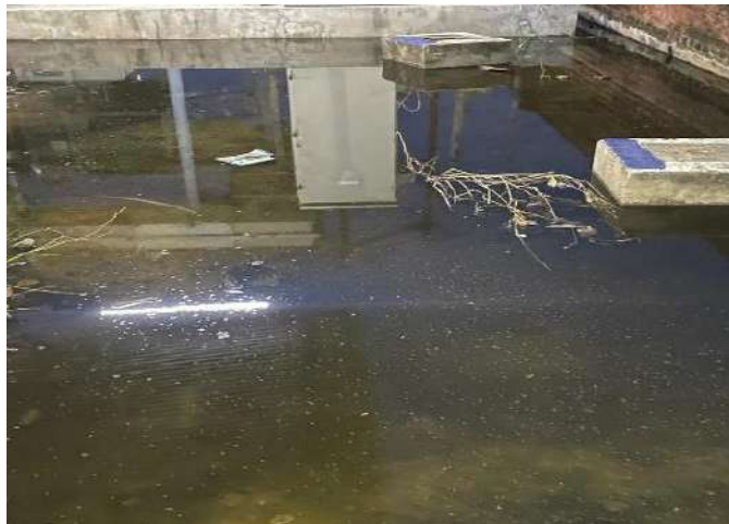
Accumulation of contaminated alkaline water within premises.
