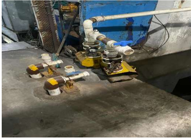
Removal of pumps from RO plant.
