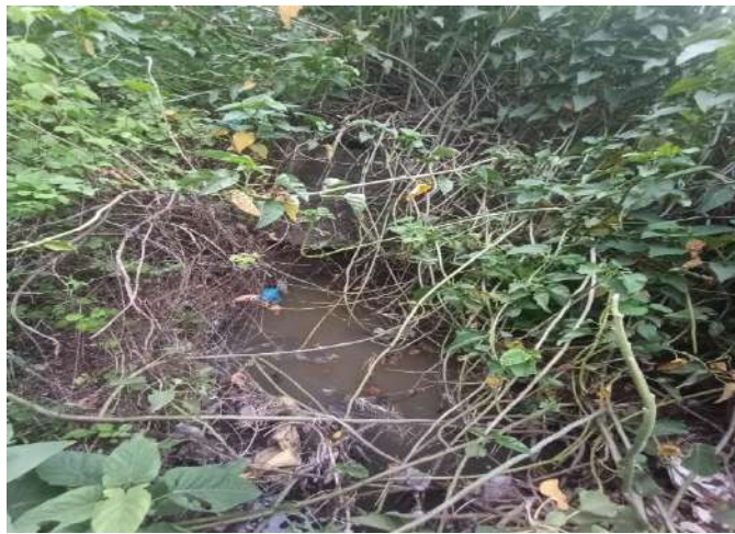
Contaminated water coming into natural drain from storm water drain of unit
